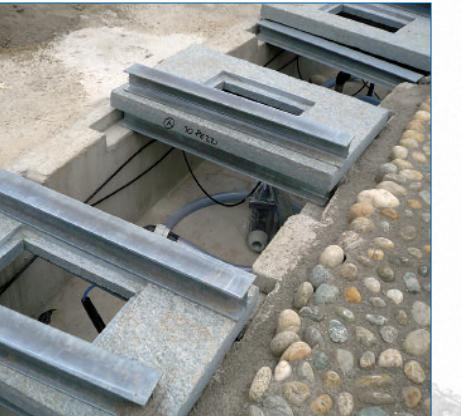
The stone slabs are supported by a steel structure, arranged so as not to interfere with the equipments.
